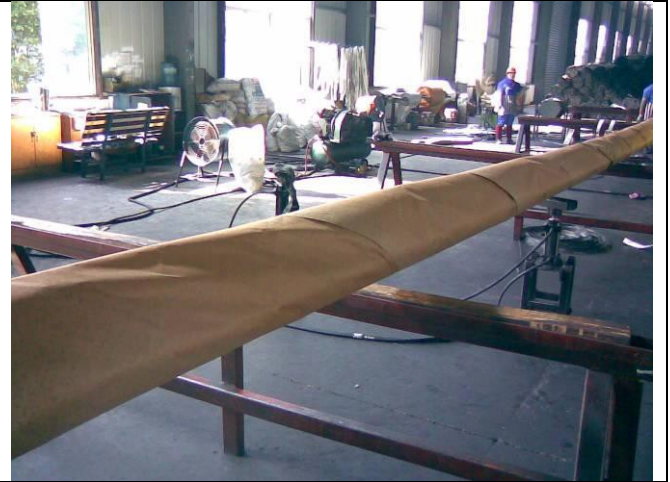
The first wrapping: Moistureproof paper
