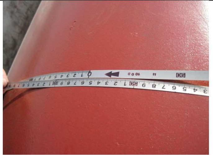
Measuring OD of pipe body
