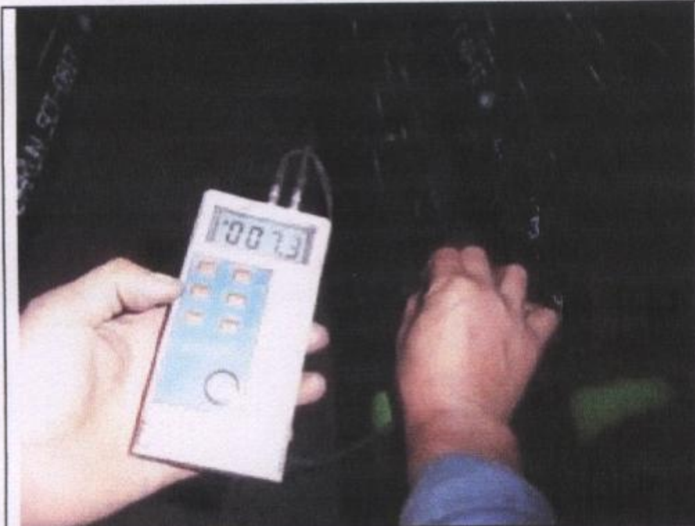
Wall thickness check.
