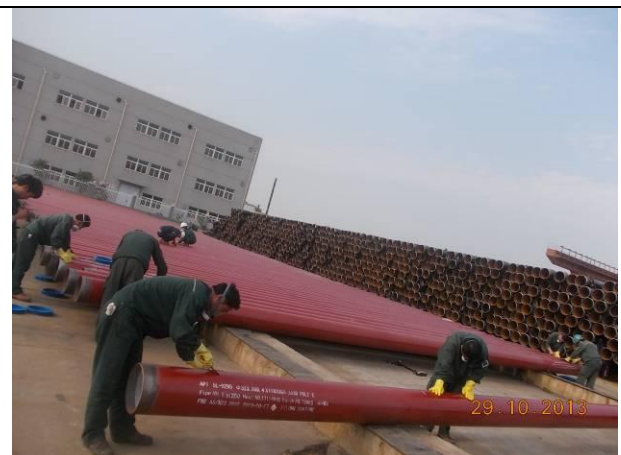
Clean the surface
