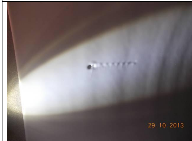
Pits were found
