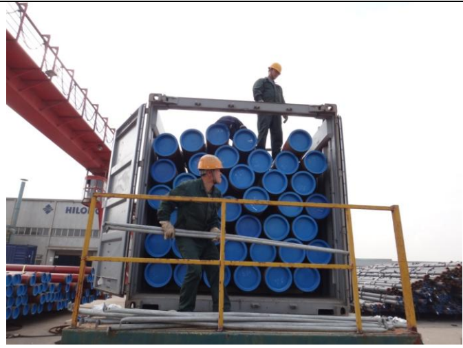
Workers passing the steel beams for top-supporting
