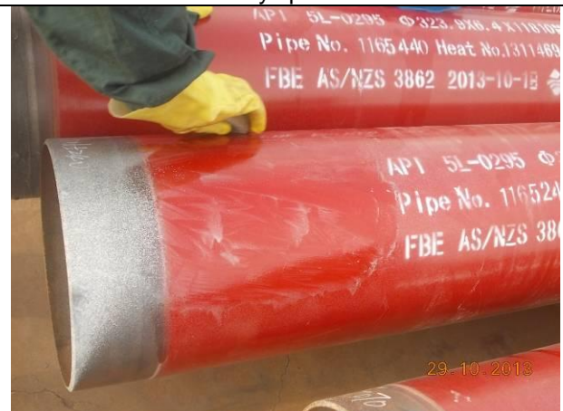
Clean the surface
