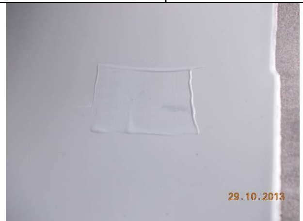
After repaired (need grind smooth)
